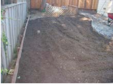
1050Acacia-070506-34__back-fence-low-retain-wall-from-SW -corner_reduced.jpg 89K
